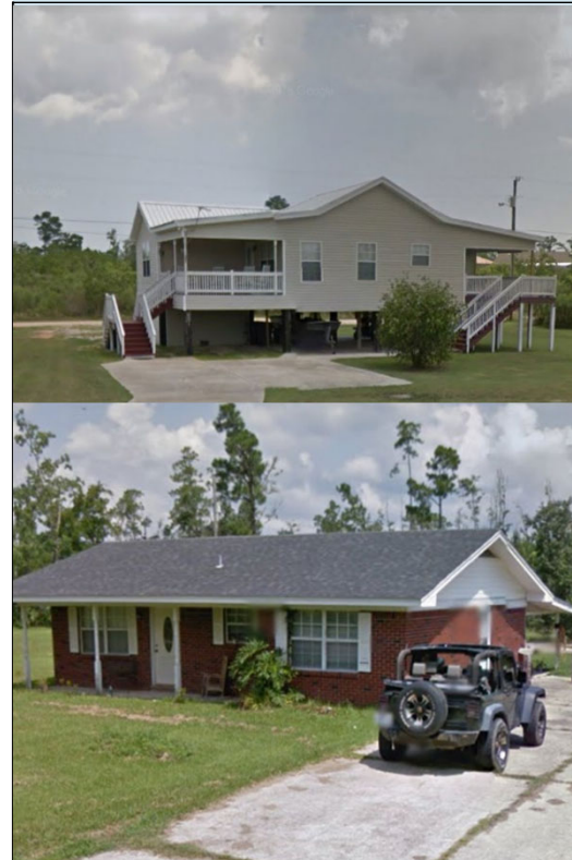
Example of the types of homes selected and mitigated under Swift Current in Mississippi.
