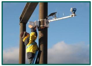
A state-of-the-art tide gauge is installed at the Hampton Fire Rescue Pier on Hampton Harbor by scientists from UMASS Boston, center for Coastal Environmental Sensing Networks (CESN) (Source - Coastal Adaption Workgroup [CAW])
