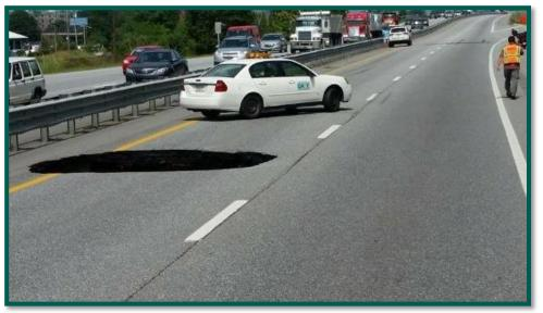
In August 2015 a 20 foot wide by 25 foot deep sinkhole appeared in Concord on Interstate 93 North between Exits 13 and 14. The cause was due to a culvert that dated back to the 1950s letting go due to its age and significant rain received the night before the collapse. (Source- NH DOT)
