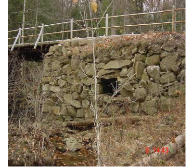
Stone Box Culvert
